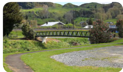
Walkways and bridges have been formed across the Mangaokewa Stream
